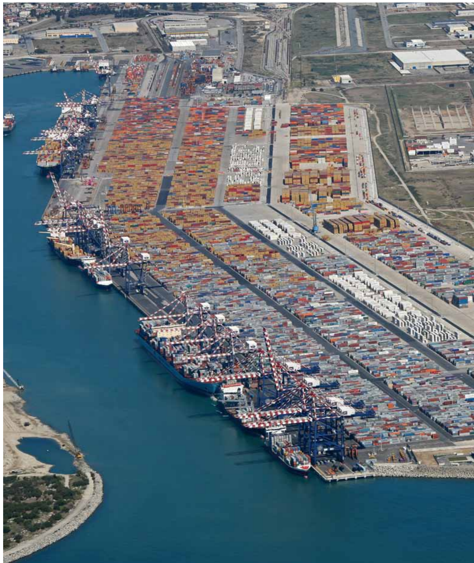
Fit for the future: the Medcenter Container Terminal in Gioia Tauro, Italy.
